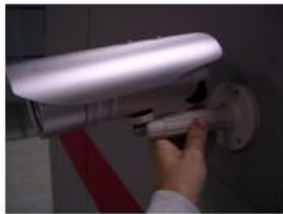
5. Install the camera onto bracket and remove sunshield
